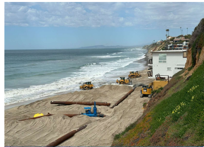
Phase III Construction & Monitoring
