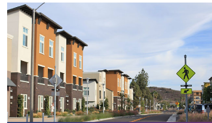
Armorlite Complete Street Corridor
