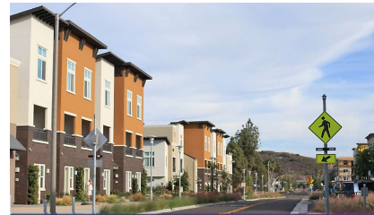
Armorlite Complete Street Corridor
