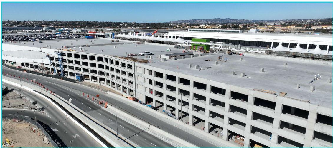
Stage 2 of Terminal 1 Parking Plaza Opened on June 13 (+2,400 stalls)
