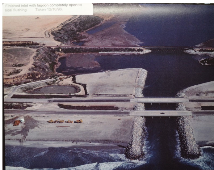
Figure 1- Rock Jetties Protecting Lagoon from Inlet Closure
