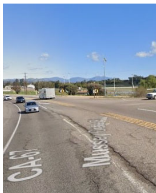
Mussey Grade Rd Intersection Safety Improvements
