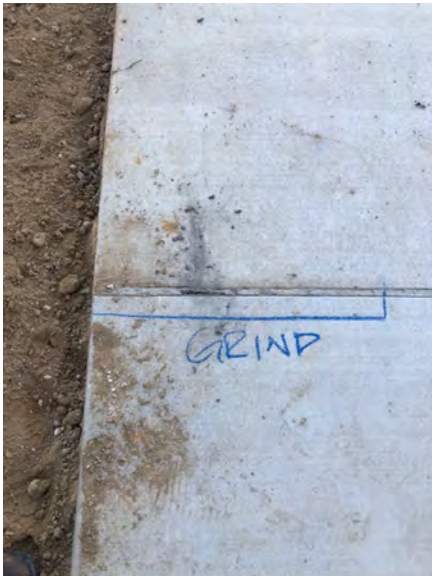
Punchlist walks are ongoing to include marking areas for repair (left), slope and dimensional verifications (center), and testing (right – cable handrail tension test)
