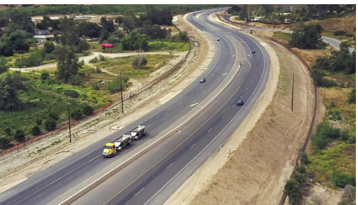
Shoulder Widening Project that widens pavement on the side of a freeway for safety in case of emergencies.
