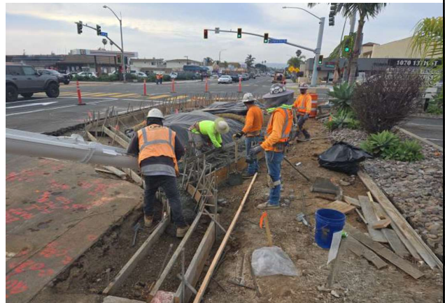
Placing concrete for trench drain system
