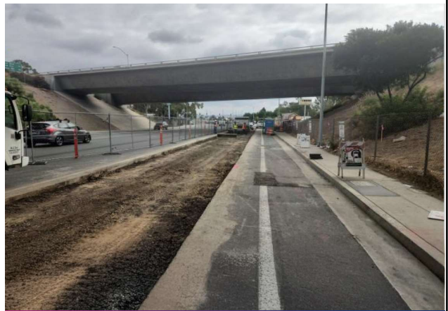
Subgrade preparation Saw-cutting existing pavement on Beyer Blvd at on Beyer Blvd at Iris Ave.
