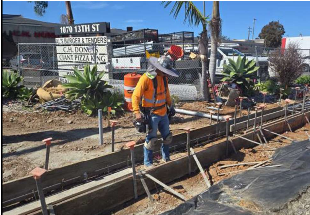
Setting rebar for trench drain system
