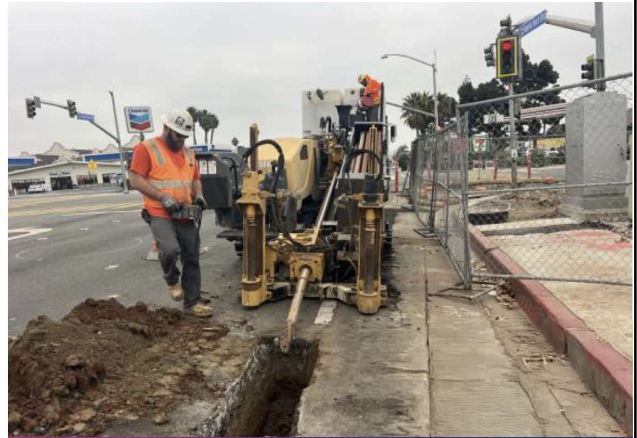
Installing traffic signal conduit at 13th St and Imperial Beach Blvd.
