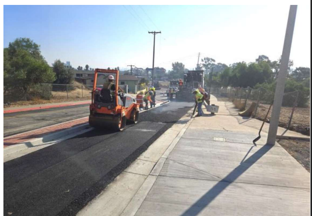
Placing asphalt concrete pavement for new bike lane on E. Beyer Blvd. near Hill St.
