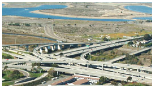
Connector A ramp that connects one highway to another.
